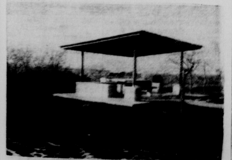
HOW ABOUT A PICNIC? —Although the weather has been a bit on the cool side lately to have a picnic, the Texas Highway Department is already preparing for warmer weather and has constructed two new picnic pavilions, like the one shown above, at the North Pocket Park.
