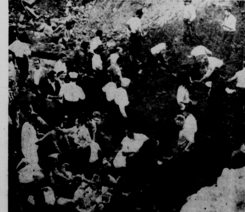
CAVE-IN TRAGEDY — SIX CHILDREN DEAD — This is a general view of the excavation site in New York where six children were killed when they were buried under tons of earth while playing in a 25-foot-deep pit.
