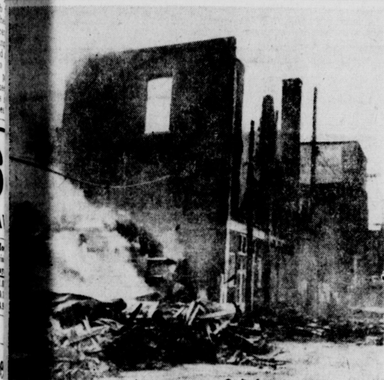
MILLION DOLLAR DAMAGE IN INDIANA TORNADO —View of wrecked business area in Union City, Indiana, after tornado and fire caused by lightning stroke consumed a square block. Damage is estimated to be in excess of $1 million.
