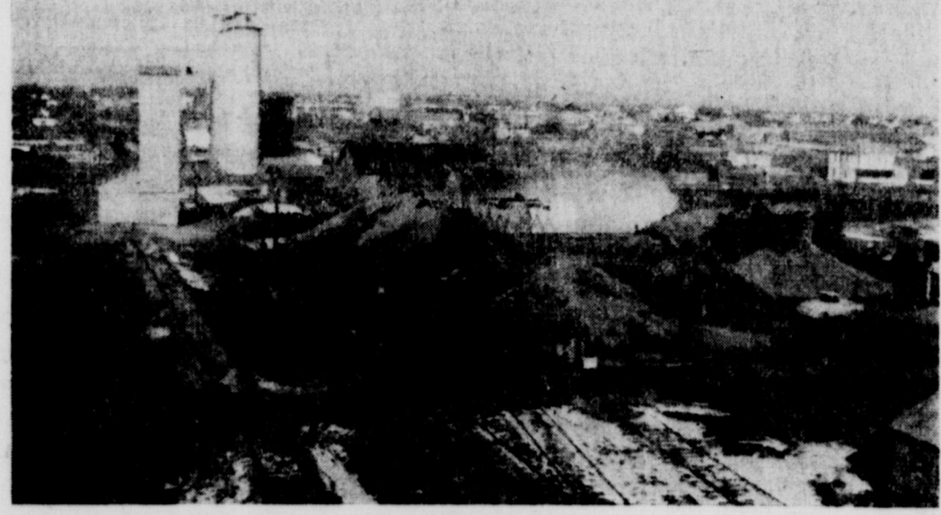
The picture above, taken by Joe Ben Roberts from the top of the Farmers Co-Operative Elevator, shows the huge piles
