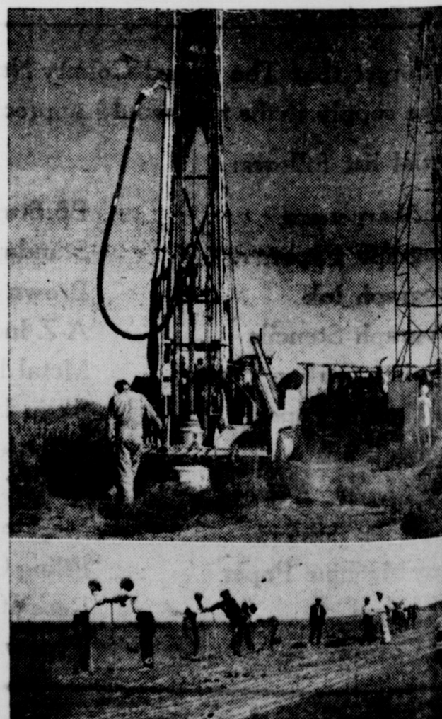
DRILLING SHOT HOLES for seismographic surveys has a long way from the hand auger days of the mid-30's, past here. Where terrain permits, today's shot hole crews use driven bits mounted on trucks. The holes are drilled for charges which, with the aid of sensitive instruments, geophysicists valuable information about the position of faults deep in the earth.
