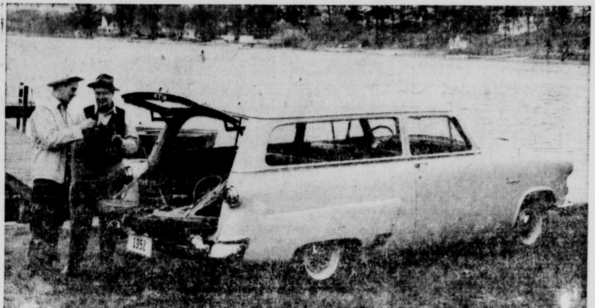
The 1952 Ford Mainline "Ranch Wagon" is a six-passenger utility vehicle for business or pleasure, in city or country. It has passenger car styling and station wagon conveniences, plus six power combinations. The Ranch Wagon is available with the Ford Mileage Maker Six or Strato-Star V-8 engine with a choice of the conventional transmission, Ford overdrive or Fordomatic—Ford's automatic transmission.
