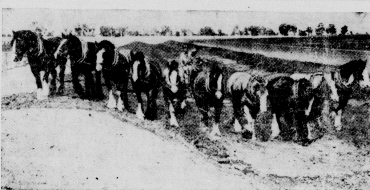
TEN HORSEPOWER IN ACTION . . . In these days of power-driven machinery, a ten-horse team is as rare as that day in June. This team is in use building an irrigation canal in the Murray valley soldier settlement, Victoria, Australia, where between 500 and 600 miles of irrigation channels are being excavated. The horses are used in preference to power machines because stamping of the horses' hoofs helps bind the soil on the banks of the channels. Notice the size and weight of the horses in this team. No wonder their feet bind the soil.
