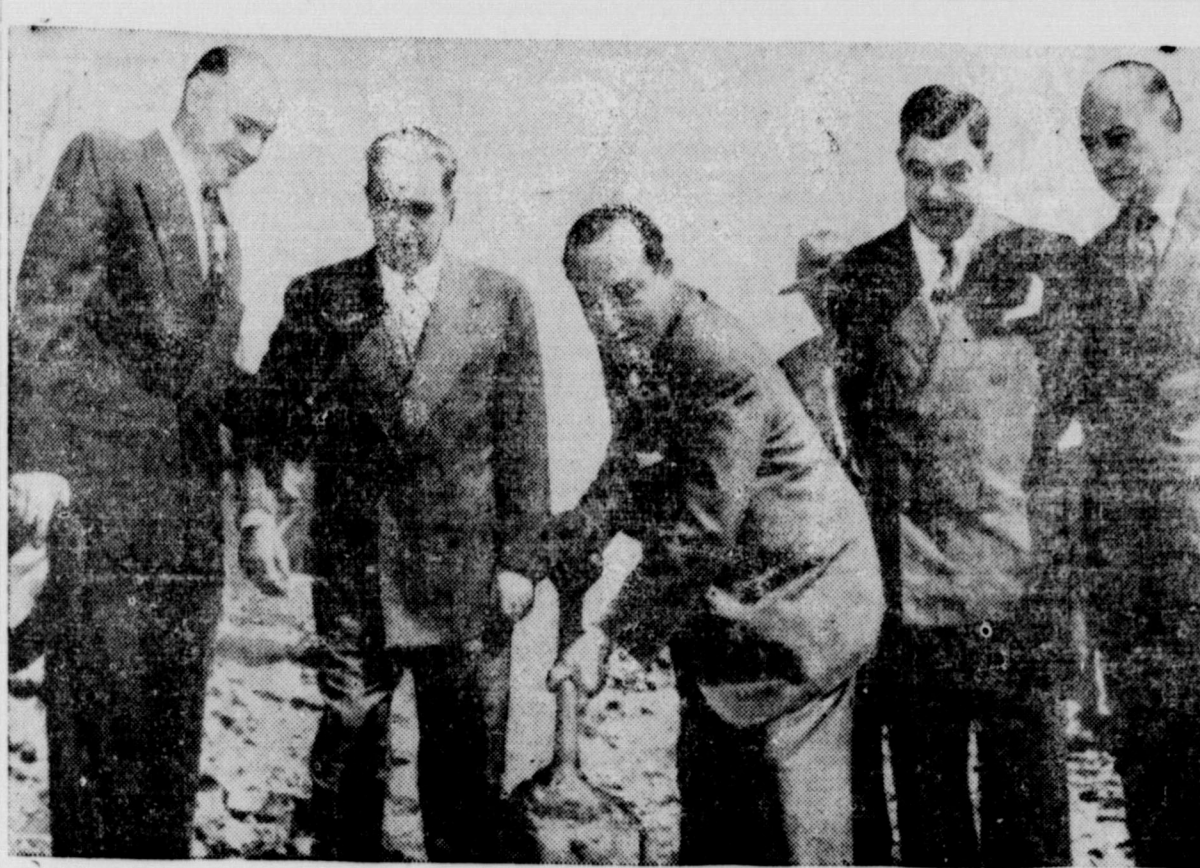
BUILDING A MONUMENT TO PEACE . . . Benjamin F. Cohen, acting secretary of the United Nations, takes the first shovelful of earth from the site of the United Nations' permanent home on New York's East river site. Cohen is hopeful that this "world capital" will succeed in maintaining peace. A $85,000,000 loan for the construction of the building was approved by congress and the building now can proceed. In the ceremonial group are left to right: Hugo Rogers, borough president of Manhattan; Mayor William O'Dwyer, Cohen, City Comptroller Lazarus Joseph and Deputy Mayor John J. Bennett.
