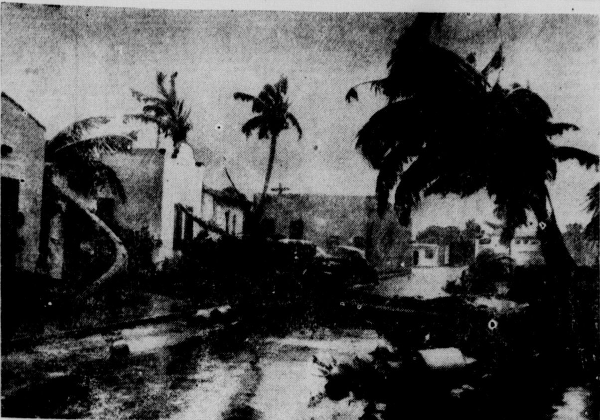
WIND OF FURY STRIKES SOUTH . . . Rolling in from the Atlantic ocean, the worst hurricane this country had experienced since 1935 slashed destructively across the southern third of Florida, leaving in its wake desolate scenes like this one at West Palm Beach. Veering out across the Gulf of Mexico, the swirling winds then struck savagely at New Orleans and Gulfport and Biloxi, Miss. Thousands in Florida and along the Gulf coast were left homeless. Damage to property and crops soared into millions of dollars.
