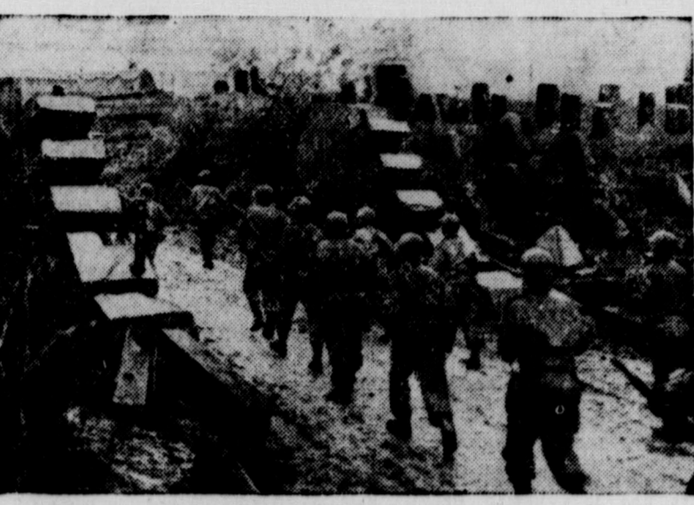
Infantrymen of the 90th U. S. division demolish part of the dragon's teeth of the Siegfried line in Habscheid, Germany, as they move to the front. Most of the barriers were made of reinforced concrete, but had little effect on the forward march of American troops. TNT and new tank guns were able to clear the way without great difficulty.
