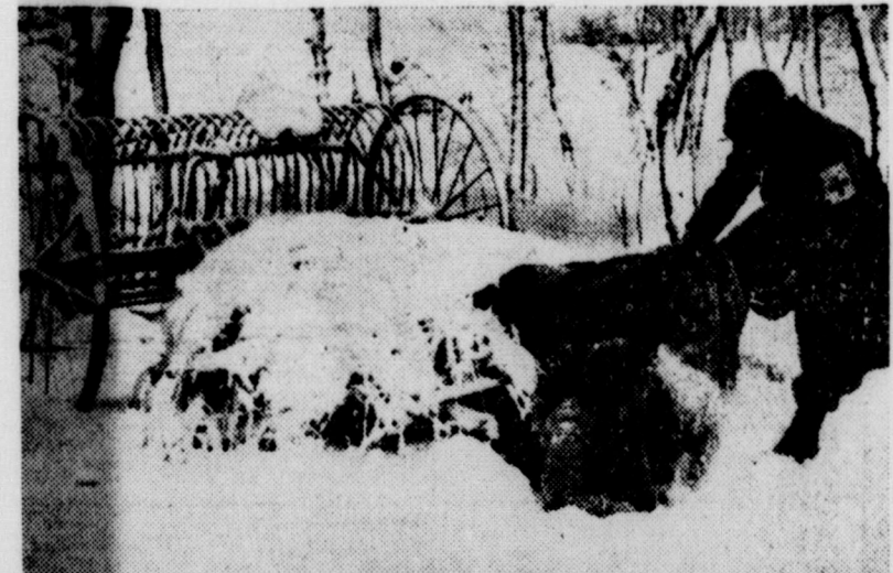
Yankee ingenuity is called into play and this "insulated" foxhole is valed on the Belgian "bulge" front. Hay and straw provide insulation against the weather. A blanket covers the door into the improvised shelter. Shafts of a hayrake provide roof supports. The tenant is Sgt. Albert Luis, Manchester, N. H.
