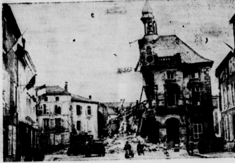
One of the freak effects sometimes achieved by high explosive bombs is seen in this photo, of a town in France, on the U. S. Third Army front. The big building at the end of the street took a direct hit and was split down the center. One-half of the building disintegrated into rubble, the other remained standing firm.
