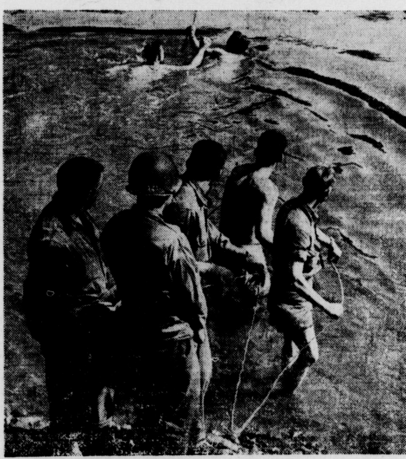
When communication lines laid across the Moselle river, France, by the signal corps battalion were broken three times, the men decided to swim the lines across the river. The signal corps work has been outstanding in this war in keeping open all lines of communication, many times under heavy fire.
