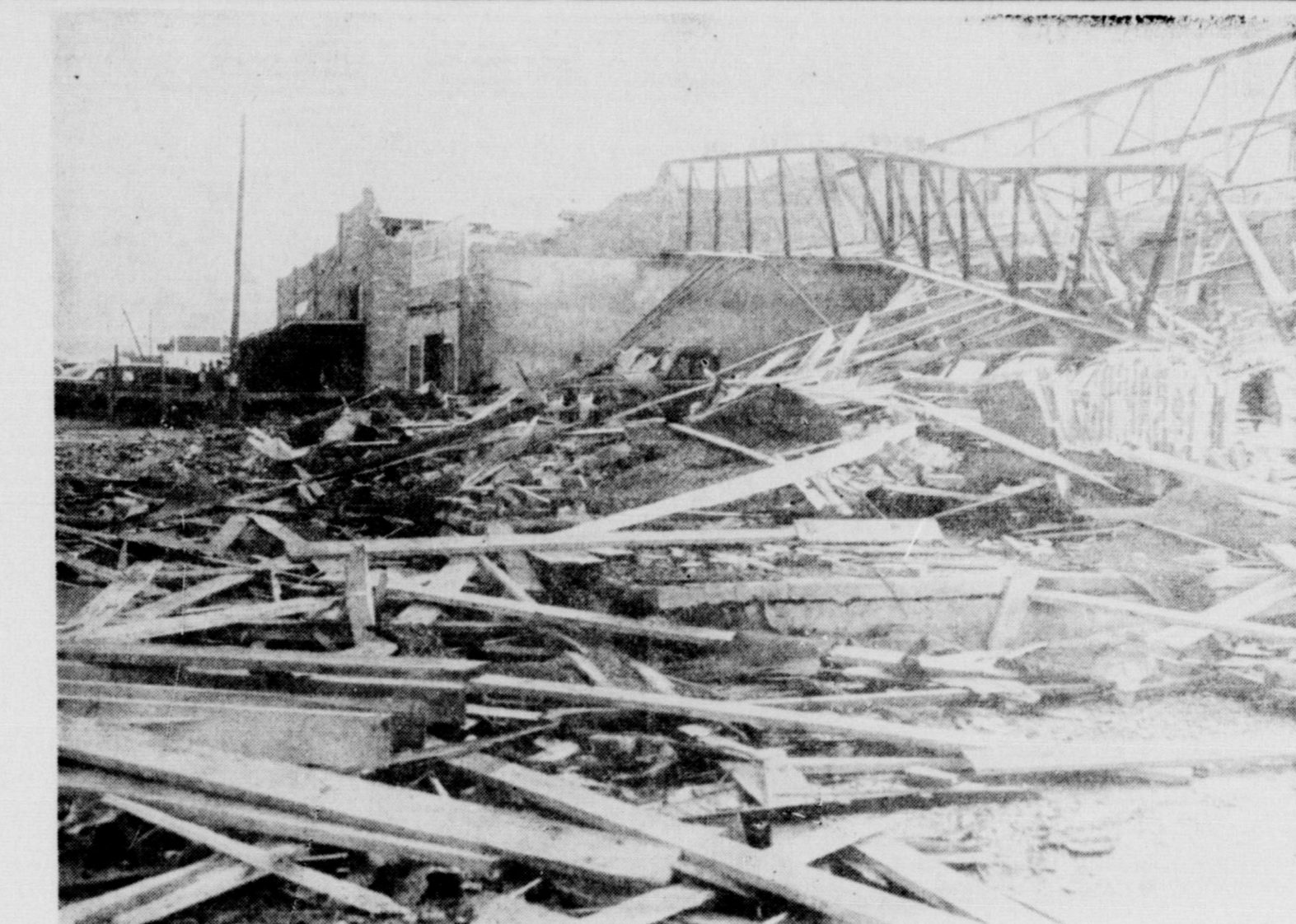
Damage to the east side of the square at Crowell is shown in the picture, made just as workers started clearing the wreckage. The Borchardt Chevrolet Company is shown in the foreground, with a number of new cars and trucks covered. Next in line is an auto supply store, The Foard County News, the first auto station and on the corner, a filling station that was converted into a cafe, supplied with food sent from neighboring towns. (Reporter-News Photo by Harry Holt)
