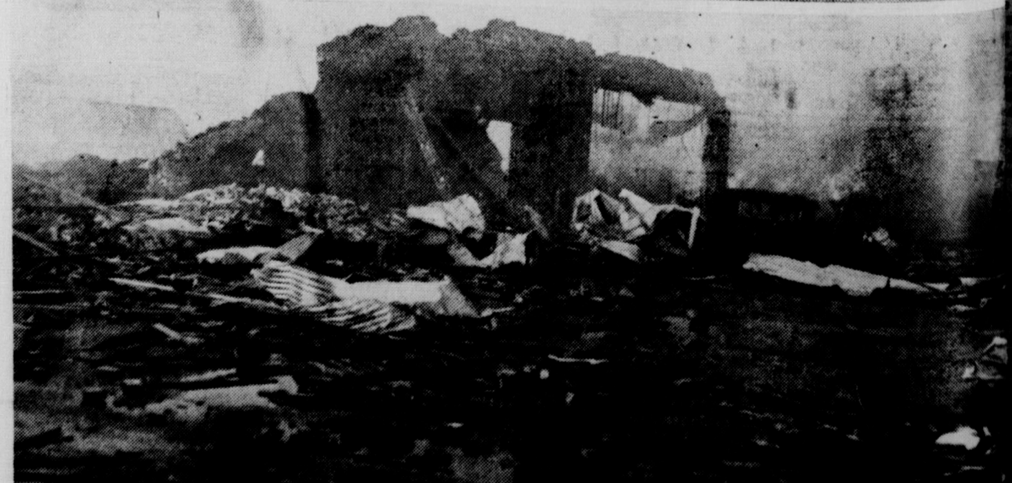
This was all that remained of Crowell's post office Wednesday morning after the town of 1,800 persons had been virtually leveled by cyclonic winds, a torrential rain and a sweeping fire. All that was left of the post office was about half of the structure which is held above by Cadet J. P. Kern, Victory Field, Vernon, and G. B. Neal, rural mail carrier at Crowell. Neal said loss is shown at the right as a brick wall toppled into the flames. For many hours the fire provided the only light in the stricken city. Emergency lights were connected to batteries and car lights used for rescue work. The remains of a beauty shop, a grocery post office, an office building and a hardware store, were leveled by wind and flames, are shown. Witnesses of the fire said flames shot out from one of the larger buildings immediately after the roof crashed. After an all-night spreading fire, firemen from a half dozen North Texas battalions were called in to help control the blaze under control shortly after dawn Wednesday. A stiff wind throughout the dark hours added to the battle.
