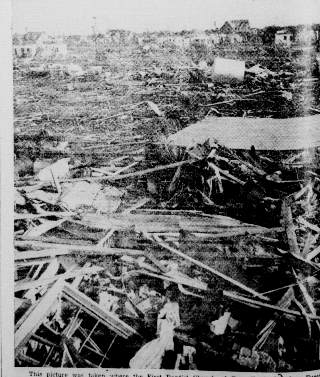
This picture was taken where the First Baptist Church of Crowell stood before Tuesday night tornado transformed it into a pile of rubbish. This view is looking north from the church site. Mrs. Alton Bell, center, is looking through the debris for some of her possessions.
