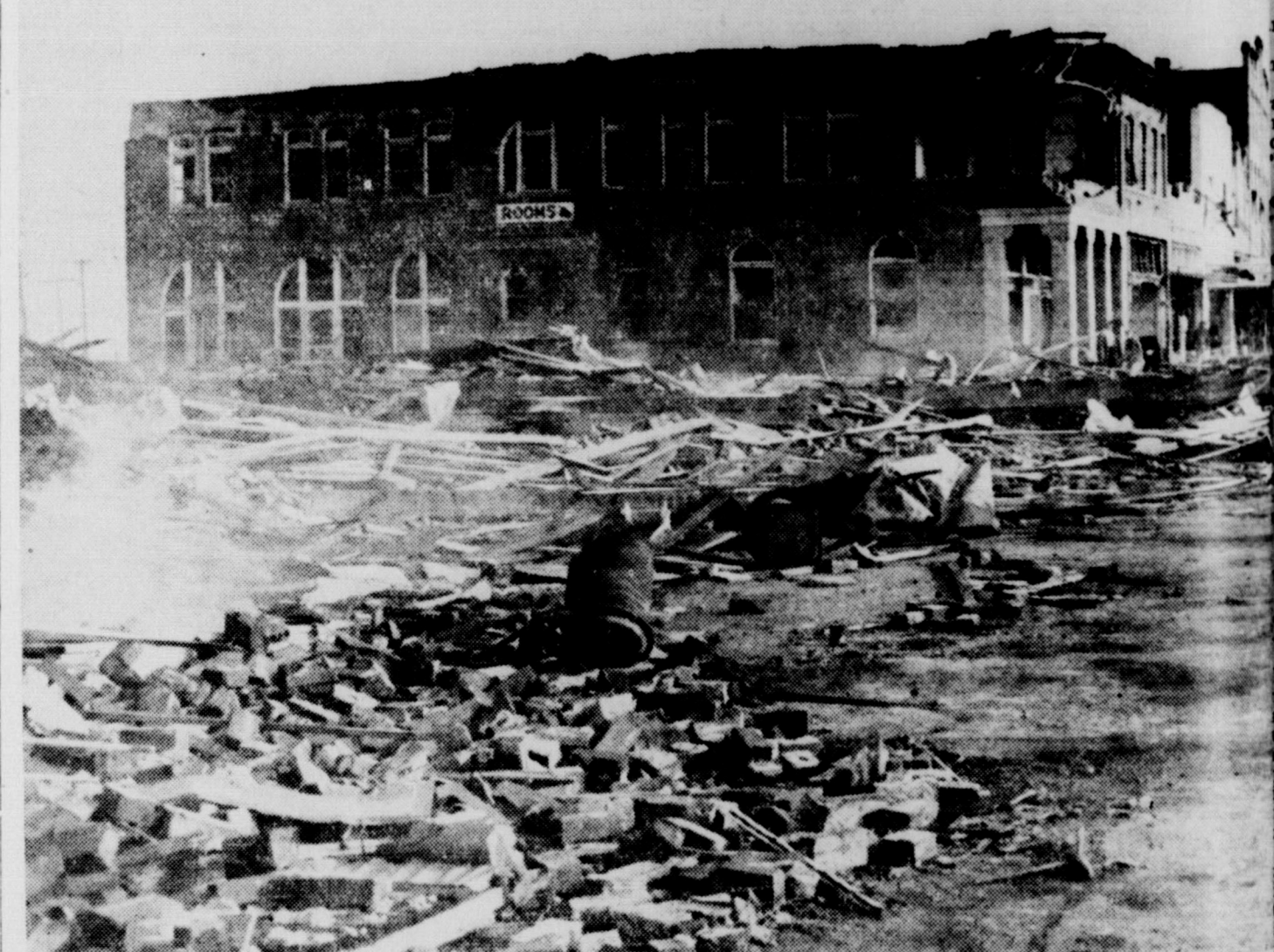
The main streets of Crowell were littered with bricks and debris southwest corner of the square, the building seemed Wednesday morning. In the scene above, looking north from the ploded with terrific force.
