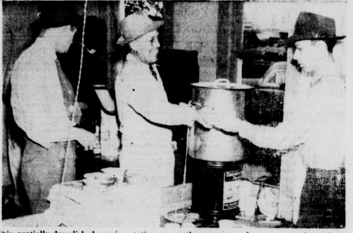
This partially-demolished service station on northeast corner of square served as "distribution center" for coffee and sandwiches sent from neighboring towns. A worker is shown receiving his sandwich.
