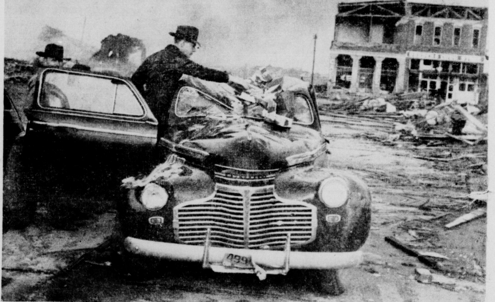
It rained bricks in Crowell Tuesday night for about 20 minutes and then hail stones almost as large as bricks fell, said Alfred Eddy, explaining the battered condition of his car. These bricks being re-
