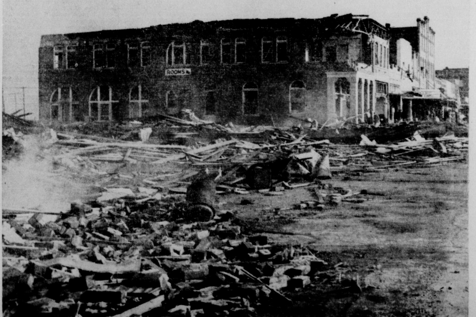
The main streets of Crowell were littered with bricks and debris Wednesday morning. In the scene above, looking north from the southwest corner of the square, the building seemed to have exploded with terrific force.
