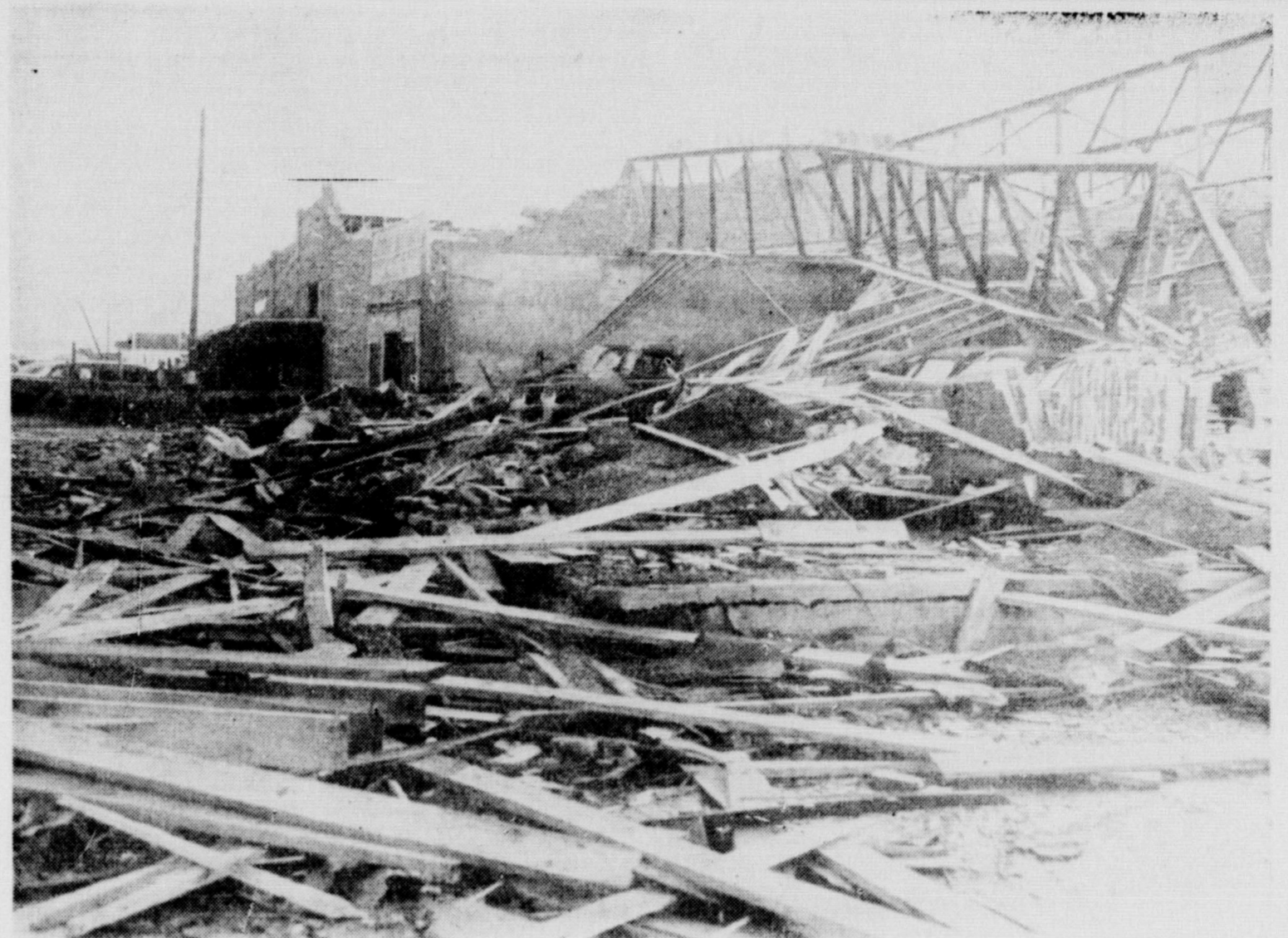
Damage to the east side of the square at Crowell is shown in the picture, made just as workers started clearing the wreckage. The Borchardt Chevrolet Company is shown in the foreground, with a number of new cars and trucks covered. Next in line is an auto supply store. The Foard County News, the first aid station and on the corner, a filling station that was converted into a cafe, supplied with food sent from neighboring towns. (Reporter-News Photo by Harry Holt)
