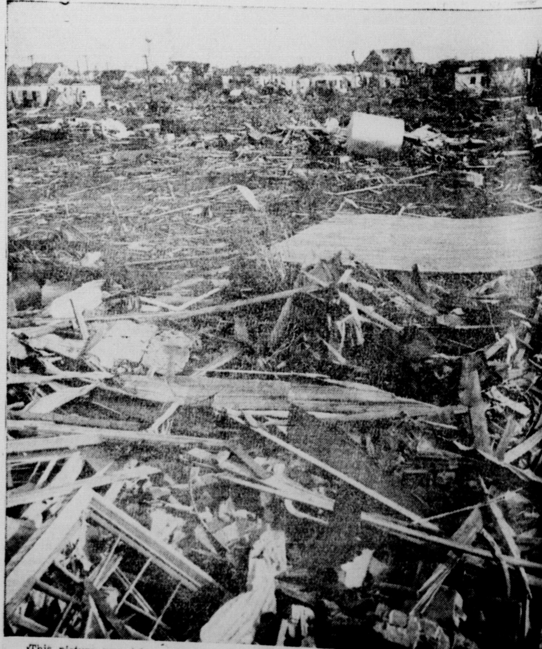
This picture was taken where the First Baptist Church of Crowell stood before Tuesday's night tornado transformed it into a pile of rubbish. This view is looking north from the church. Mrs. Alton Bell, center, is looking through the debris for some of her possessions.
