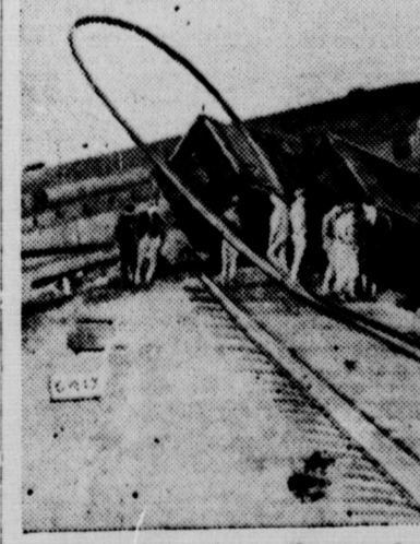
This photo shows the wrecked locomotive, tender and car of the streamlined railroad train that struck a truck near Dallas, Texas. Note the rail twisted and uprooted 30 feet in the air by the impact. Two were killed as a result of the accident.
