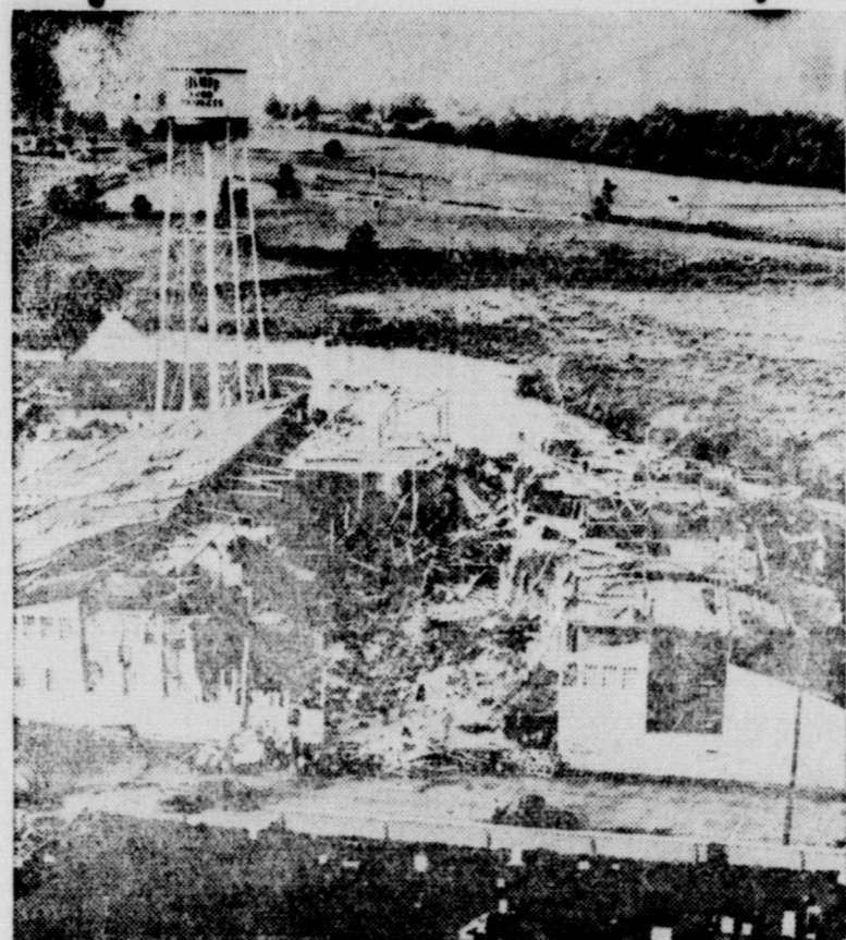
Shown here are the ruins of a cannery factory at Swedesboro, N. J., after a tornado had ripped it to pieces. George Hemple, of Swedesboro, was crushed to death when a 150-foot steel stack at the cannery fell on and smashed the truck in which he was sitting. Eighty others were injured in the cannery. Other sections of Delaware and New Jersey suffered damage from the storm.
