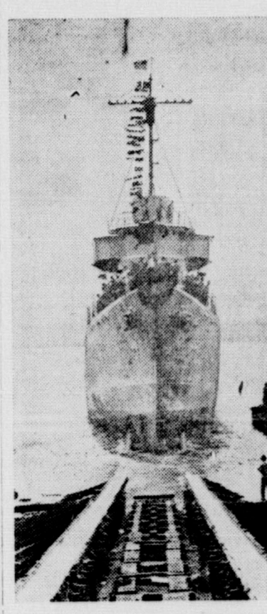
The U. S. S. Ellyson slides down the ways at Federal ship yards, Kearney, N. J. It took the water a short time after the U. S. S. Bristol, which was first out in the twin launching. Both ships were built in record time.
