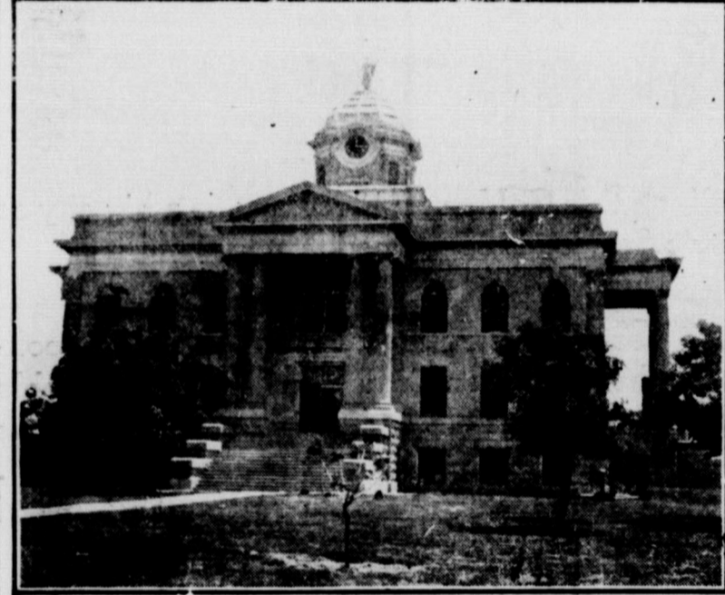
Pictured above is Foard County's present court house. It was completed in 1910.
