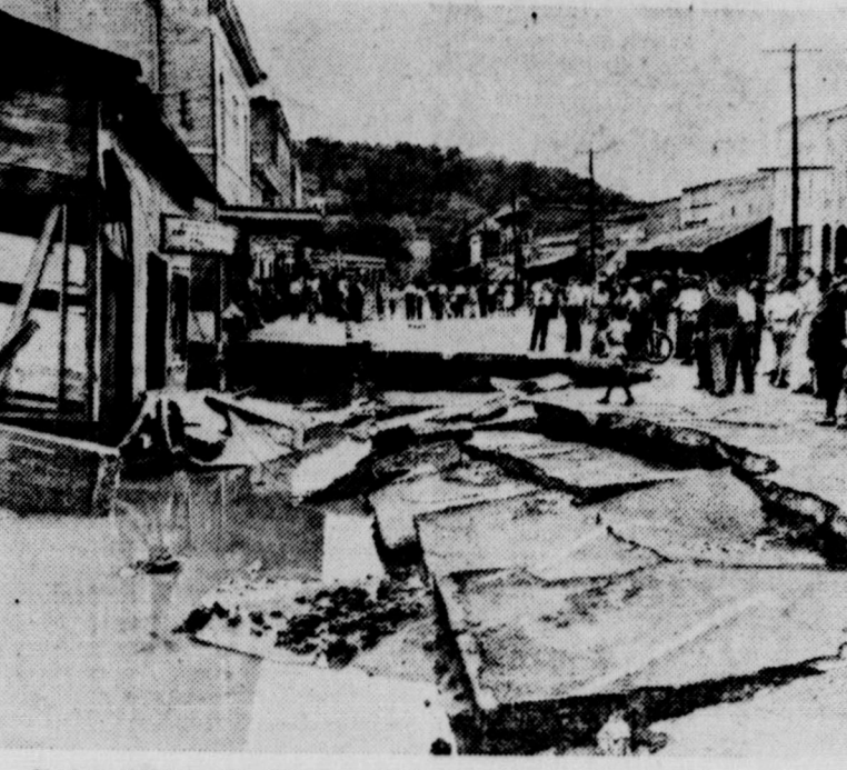
Undermined by flood waters from a swollen tributary of the Alabama river, this section of the Prattsville, Ala., main street collapsed, halting traffic through the business district. Floods were caused by heavy rains, and though there was no loss of life, more than 2,000 persons in the southern part of the state were forced to flee their homes.
