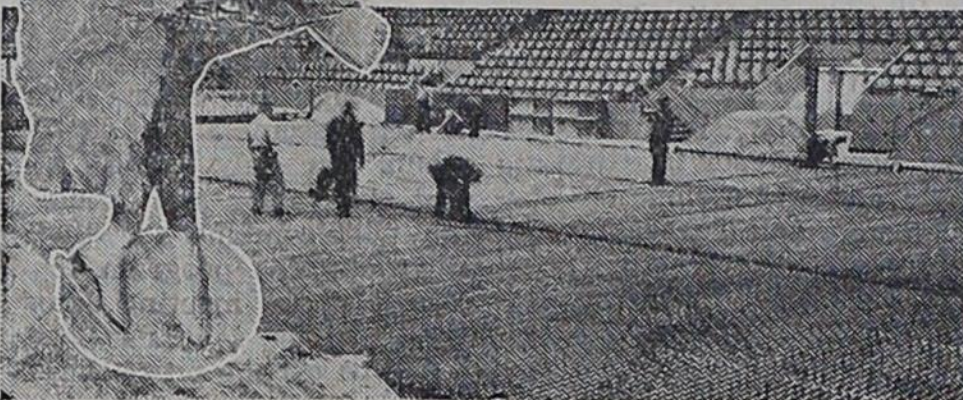
STAGE FOR EACH SHOW, carried about the nation in trailers powered by International truck-tractors, is 9,600 square feet of piping. Brine is circulated through the piping which is then covered with water. Freezing action quickly creates smooth skating surface.
