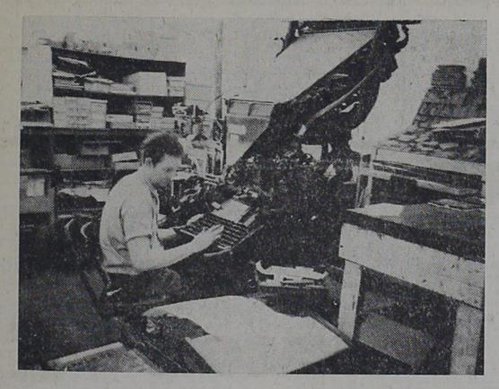
This is our typesetting machine, the Linotype, which was purchased in 1924 by J. A. Kennedy and still turning out the work, setting most of the type for the newspaper. A few repairs in time keep this dependable piece of machinery going. Wallace L. (Wally) Park is the operator.
