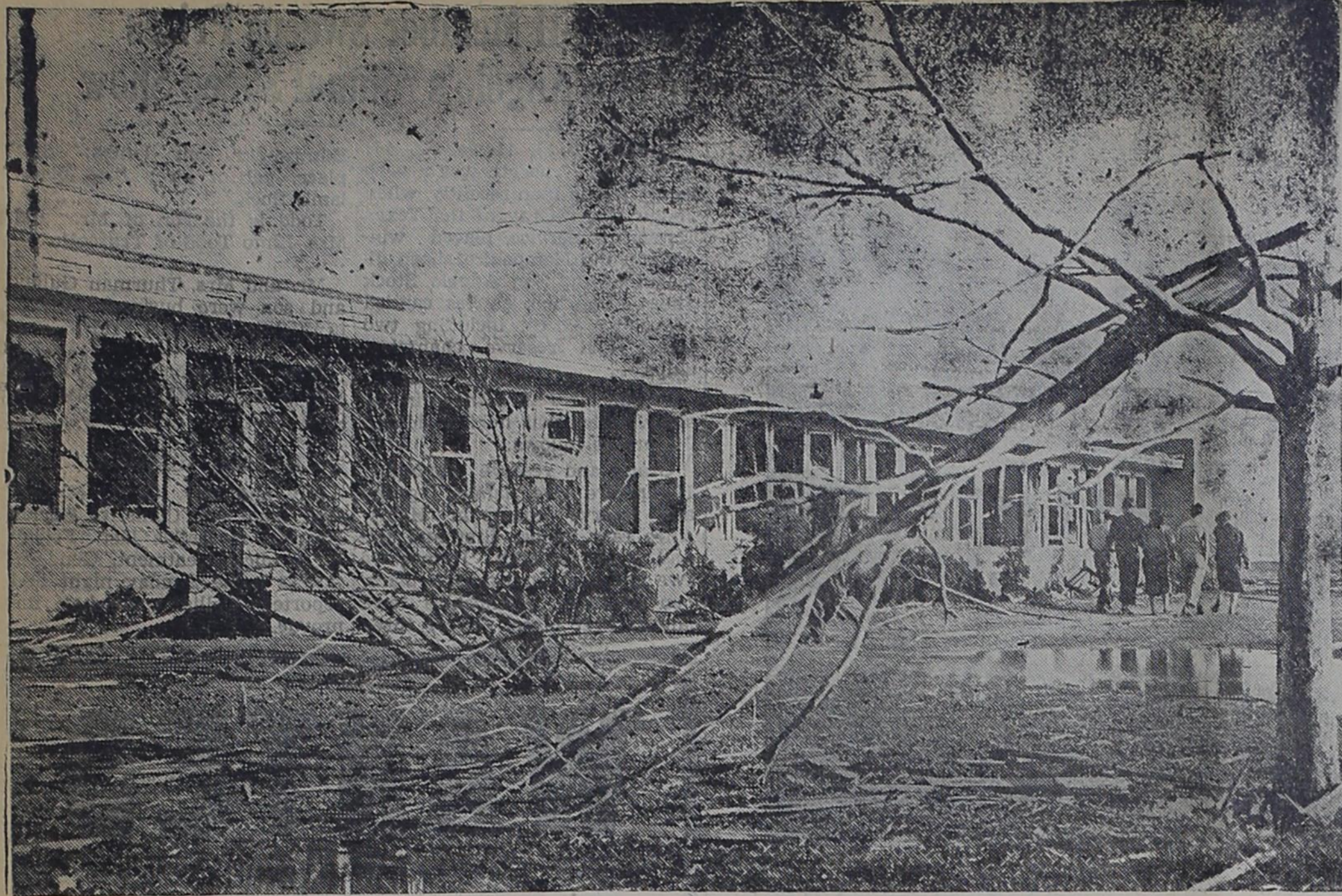
WHERE THE STORM FIRST STRUCK—As a death-dealing tornado roared out of the southwest Friday afternoon, the first building to be struck was the Knox County Hospital, shown
