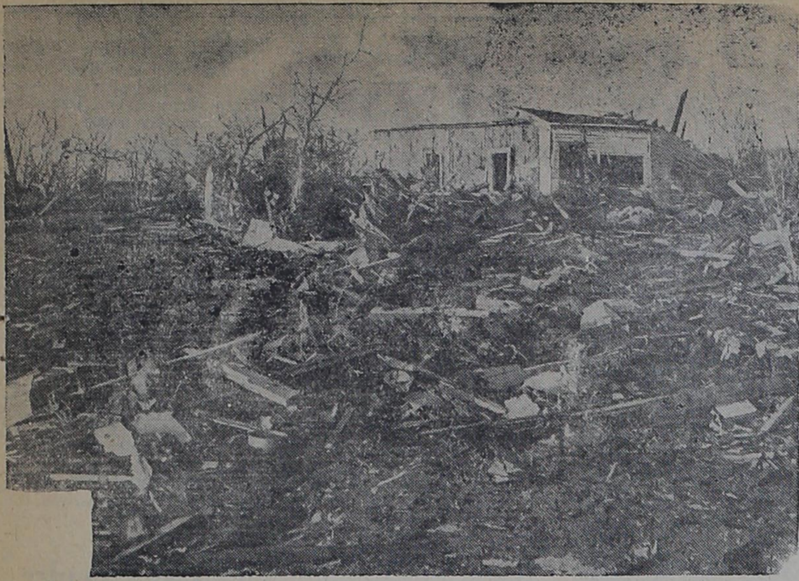
TWO DIED HERE—All that remains of 10 houses in this square block is the shambles shown at the rear. Two women trapped in a dwelling that formerly stood
