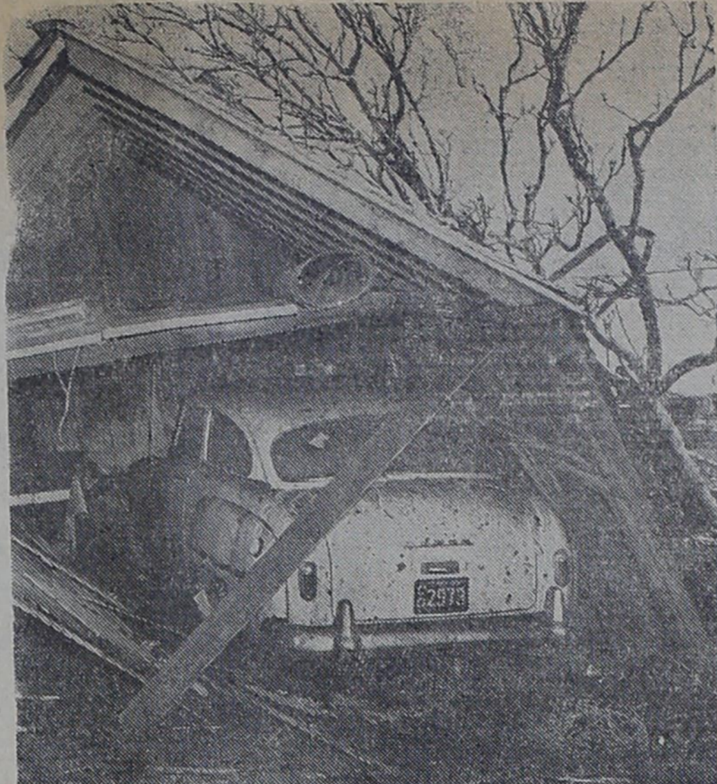
CAR SLIGHTLY DAMAGED—Miss Mary Parsons, who worked at the clinic in Knox City, saw the tornado coming and rushed her automobile to the garage.
