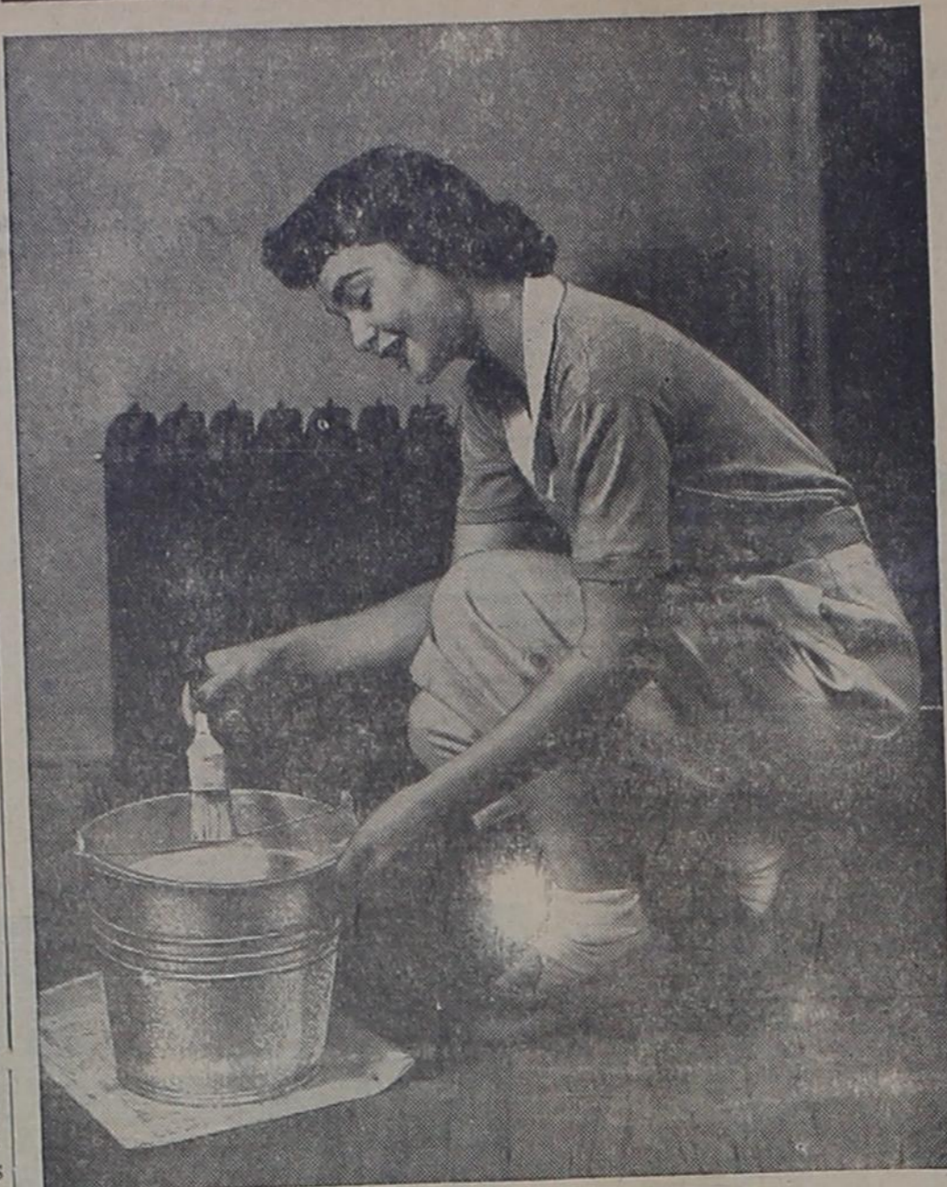
Make radiators less conspicuous by painting them the same color as walls. To avoid splattering paint, string a piece of wire across the mouth of a galvanized steel paint pail. The wire may be attached as shown. Simply pat the brush against the wire to remove excess paint.
