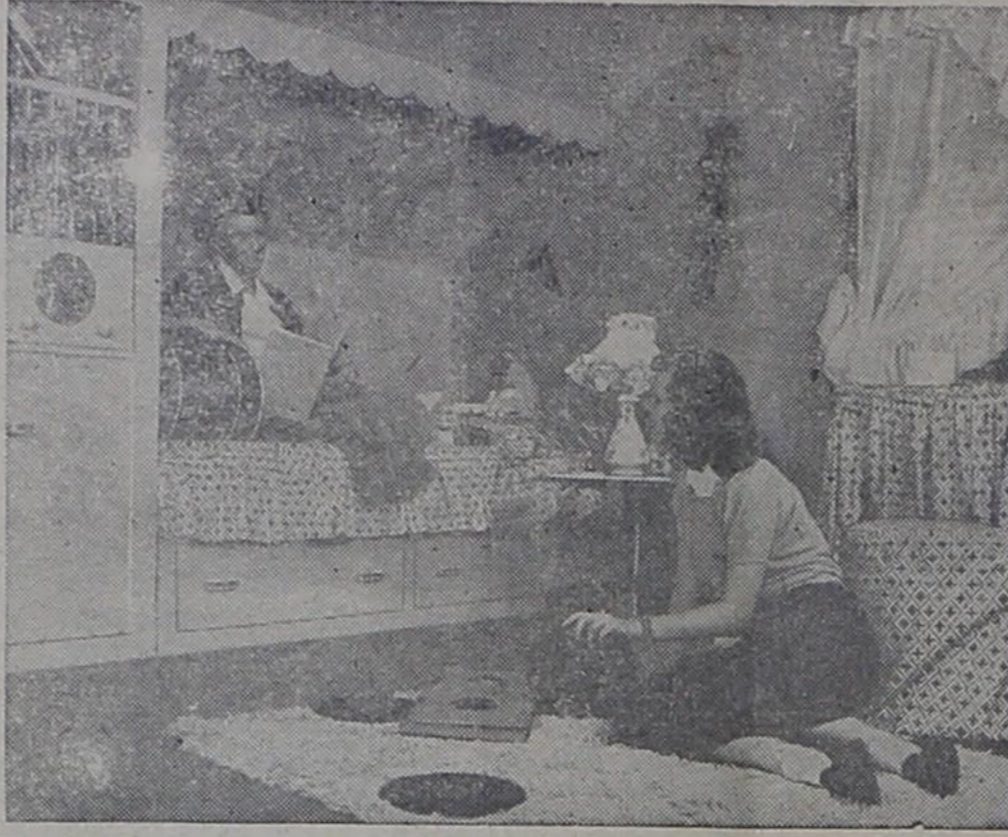
A comfortable, attractive room in the attic will please the adolescent, especially if it is furnished for multiple purposes of work, recreation and sleep. In the room shown, the open studding was covered with Masonite Panelwood, a material which can be painted or papered and which stands lots of abuse. Note the storage drawers under the built-in bunk, the neat arrangement of albums over the closed record player, and the storage cabinet.
