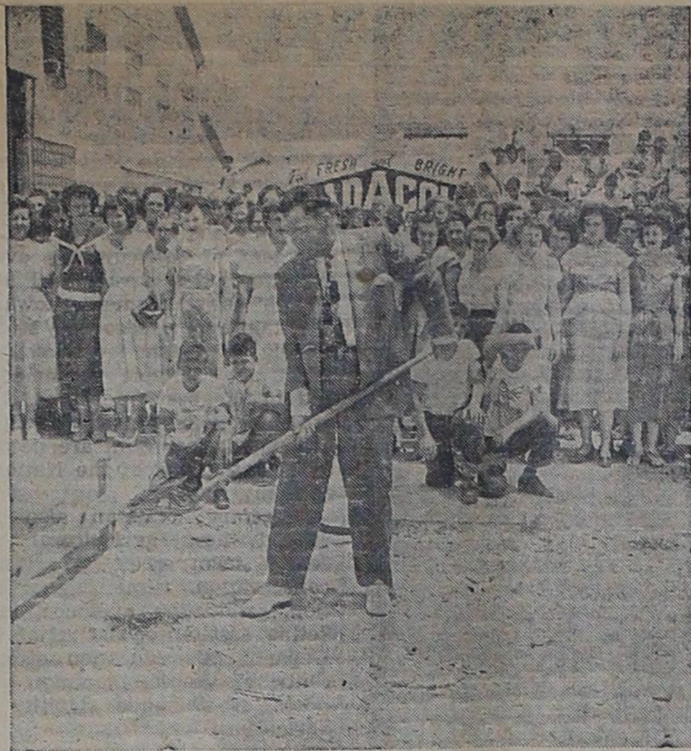
Senator Dudley J. LeBlanc, creator of famous HADACOL is shown above breaking ground for the new HADACOL factory now being built alongside the present plant in Lafayette, Louisiana. This new building will be 80x235 feet, two stories, steel and concrete construction. The remarkable growth of HADACOL has forced the immediate construction of this new building. Only last spring Senator LeBlanc opened the present HADACOL plant and now less than a year later, HADACOL requires a 100% increase in factory space.
