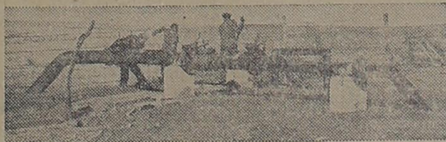
BEHIND GAS SERVICE there is something to build, paint, or repair every day, oftentimes in remote places. Above, a crew completes a control valve installation, part of a new compressor station. In the last three years, Lone Star has invested over $100 per customer to assure dependable service. Yet, you enjoy conveniences and comforts of natural gas service for a year around average of less than 15c a day.
