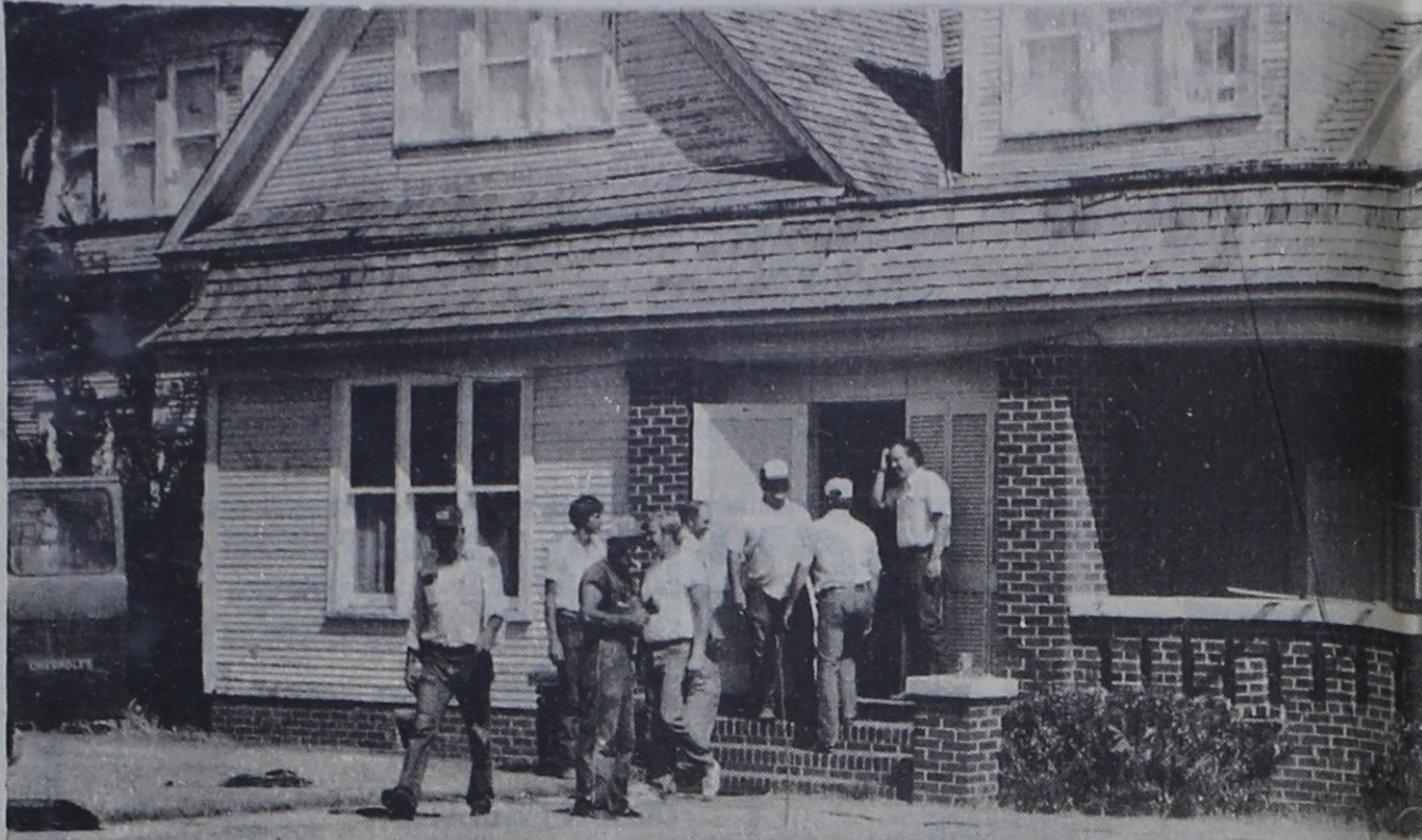
A SKILLET FIRE filled the Bill Longan home with smoke one night last week, and Munday volunteer firefighters were called to ventilate the house. A spokesman for the department, of which Longan is a member, said nothing in the home burned and no damage was reported.
