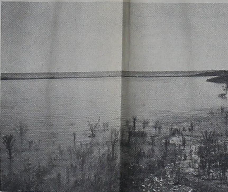
LOOKS LIKE A LAKE: This shows water in the reservoir basin. Although it takes on the appearance of the lake when looking toward the dam, water has not yet reached the dam.
