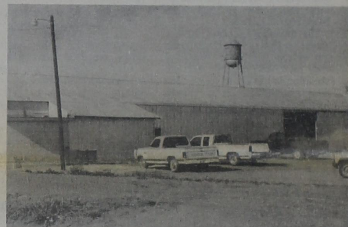
THE NEWLY REMODELED Knox County Livestock Show Barn stands ready for its inhabitants this weekend during the annual junior livestock show. Members of the young farmers group have made extensive improvements and additions to the building with the help of donations from local individuals and businesses. The facility was originally the Colville and Wilson potato shed building, and is located in the southeast part of Munday.
