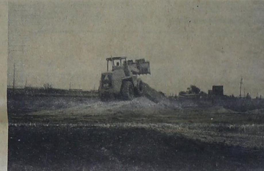
ANOTHER PIECE of heavy machinery aiding in the construction work.
