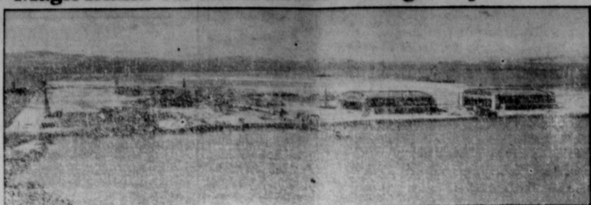
The 430-acre site of the Golden Gate International Exposition shown above is literally a magic island for it was made of material dredged up from the sea. After the exposition in 1939 it will be transformed into a fine municipal airport.
