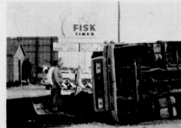
HAY ON HIGHWAY ---- This semi-truck, loaded with chopped hay overturned Thursday morning early at the detour where construction is underway on Highway 84. Rhea Bradley, engineer, points out that this is one of the most dangerous spots along the construction route on West Highway 84 out of Muleshoe. The truck belongs to National Alfalfa Dehydrating Mill. No injuries were reported. Hay was strewn over a section of the road.
