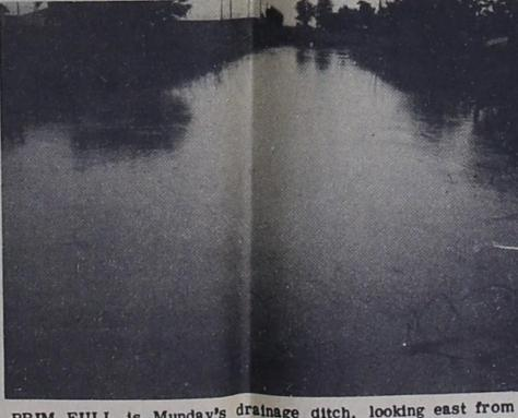
BRIM FULL is Munday's drainage ditch, looking east from Highway 277 to the railroad and showing inadequate drainage facilities under the railroad.
