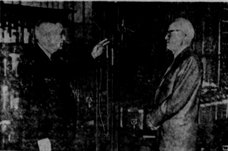
Charles Edison, son of Thomas Alva Edison and chairman of the board of McGraw-Edison Company, shows Max McGraw, president, how the famed inventor developed the first successful incandescent light bulb 80 years ago this year (Oct. 21, 1879). Arrow points to replica of the first bulb mounted on the mercury pump used to exhaust air around the carbonized cotton-thread filament. Scene is the original Menlo Park Laboratory which Henry Ford moved to Greenfield Village, Dearborn, Mich., in 1929.
