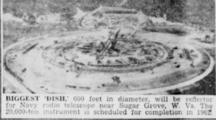
BIGGEST 'DISH,' 600 feet in diameter, will be reflector for Navy radio telescope near Sugar Grove, W. Va. The 20,000-ton instrument is scheduled for completion in 1962.
