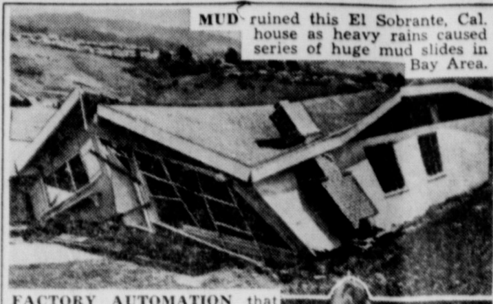
MUD ruined this El Sobrante, Cal. house as heavy rains caused series of huge mud slides in Bay Area.
