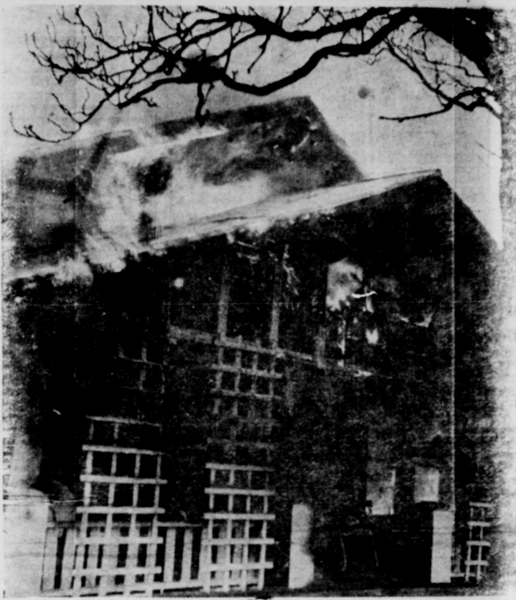
LANDMARK DESTROYED — Flames are shown shooting from the roof of the Lansford Apartments in Munday as this landmark was gutted by fire early Saturday afternoon. Quick and efficient work of the Munday Volunteer Fire Department saved nearby buildings from destruction as the high winds whipped the flames.
