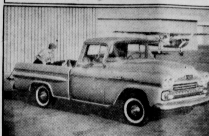
Modern sculptured styling, 50 percent more load space, and stronger construction feature the new Fleetside pickup trucks added to the Chevrolet line. The cargo area is two feet wider and slightly deeper than conventional models. Running boards and fenders are absorbed into the body. Contoured jet-pods add sculptured style and strength to side panels.
