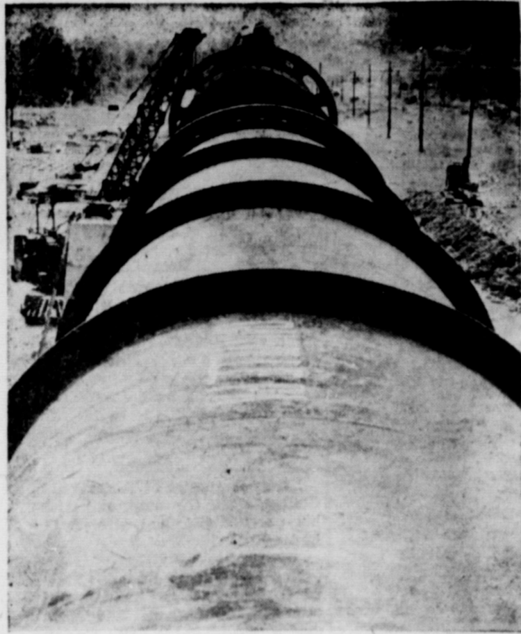
One of the world's largest single pieces of precision mechanized equipment, a 300-foot rotary kiln for the manufacture of cement, is being completed at the Texas Portland Cement Plant at Orange, Texas.
