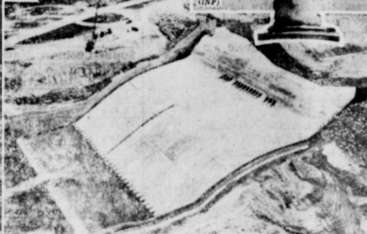
SPILLWAY of new $19,500,000 Kirwin Dam near Phillipsburg, Mo. Under test.
