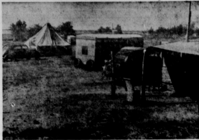
Where huge defense plants have been built near hamlets or small towns, housing is usually inadequate and sub standard. Many defense workers must live in tents, trailers and hastily built shanties like those shown here. United Community Defense Services, member agency of United Defense Fund, helps communities plan and set up basic services. UDF seeks support through Community Chest or United Fund drives.
