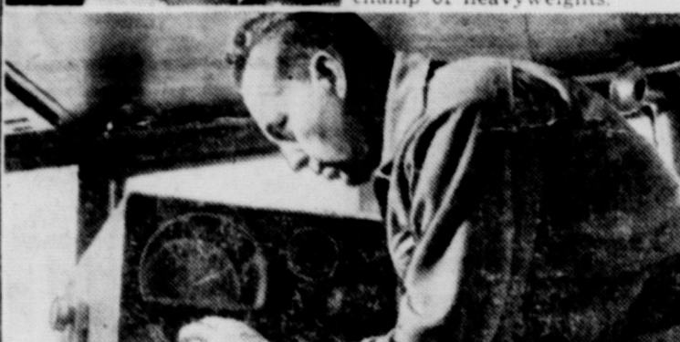
UNDERSEA TV? —New "Sea Seasar" electronic device developed by Minneapolis-Honeywell uses sound waves to help fishermen and marine pilots to "see" bottom contours, fish, obstructions, sweeping in 180-degree arcs to spot objects up to 1,600 feet away.
