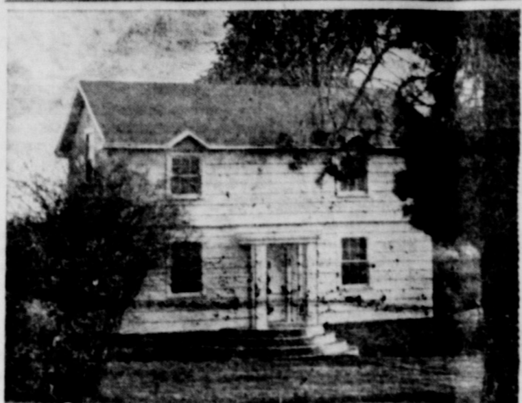
Does it pay to modernize? These pictures are a Californian's answer to the question. They show the conversion of an over-age farm dwelling (above) much the worse for wear and showing signs of obsolescence, into a trim attractive home (below). New siding of asbestos-cement shingles effected the major transformation, plus making the house more weather-tight and adding to its fire safety. Breaking the roof with tiny dormers permitted the addition of second story windows and better utilization of the living area. A modern entrance gave the final touch.
