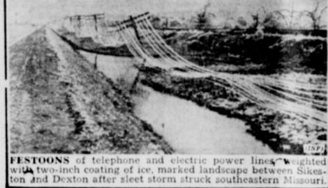
FESTOONS of telephone and electric power lines, weighted with two-inch coating of ice, marked landscape between Sikeston and Dexter after sleet storm struck southeastern Missouri.
