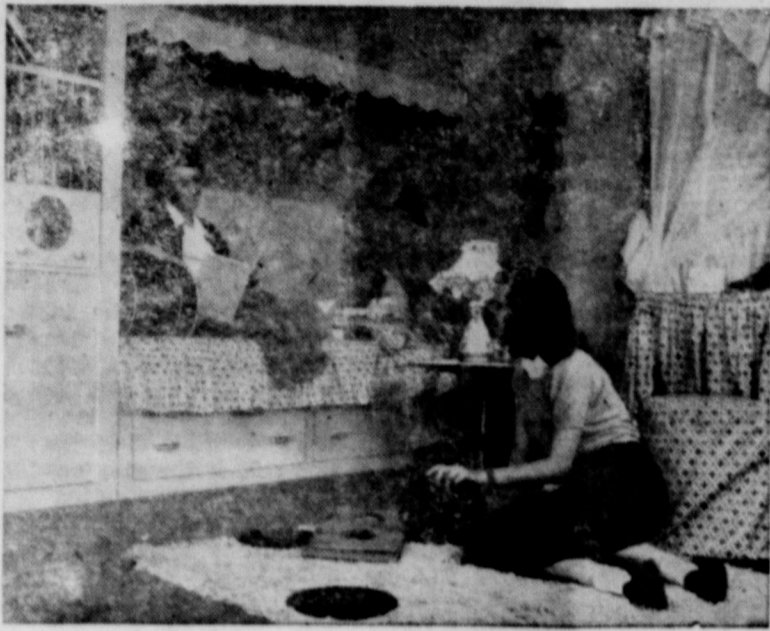
A comfortable, attractive room in the attic will please the adolescent, especially if it is furnished for multiple purposes of work, recreation and sleep. In the room shown, the open studding was covered with Masonite Panelwood, a material which can be painted or papered and which stands lots of abuse. Note the storage drawers under the built-in bunk, the neat arrangement of albums over the closed record player, and the storage cabinet.
