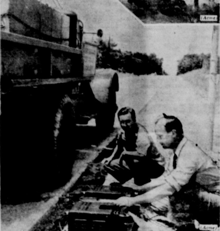
CRACKATHON—Scientific tests to measure road damage inflicted by heavy trucks are under way on this mile-stretch of highway in Maryland sponsored by 11 states alarmed over road deterioration. Laden with concrete, the trucks will travel 500,000 miles to nowhere. Here U.S. engineers check for wear and tear.
