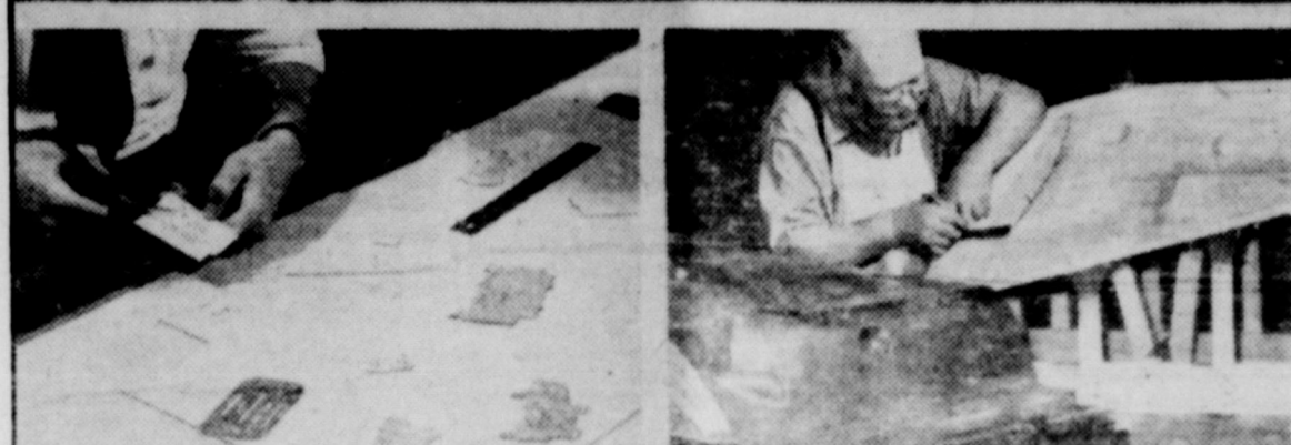
Skilled hands continue in demand in the manufacture of automobiles, despite the rise of machines. Here's evidence in pictures taken at the Chevrolet plant: (Top)—A crew positions 60 vanes of the Powerglide automatic transmission before the assembly is spot welded. (Lower left)—To plan factory layouts draftsmen cut out cross-sections of the floor area of machines at scales of precisely one-quarter inch to one foot. (Lower right)—A pattern maker cuts a wooden model that will later be duplicated in steel to stamp out thousands of fender parts.
