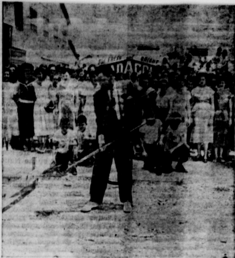
Senator Dudley J. LeBlanc, creator of famous HADACOL is shown above breaking ground for the new HADACOL factory now being built alongside the present plant in Lafayette, Louisiana. This new building will be 80x235 feet, two stories, steel and concrete construction. The remarkable growth of HADACOL has forced the immediate construction of this new building. Only last spring Senator LeBlanc opened the present HADACOL plant and now less than a year later, HADACOL requires a 100% increase in factory space.
