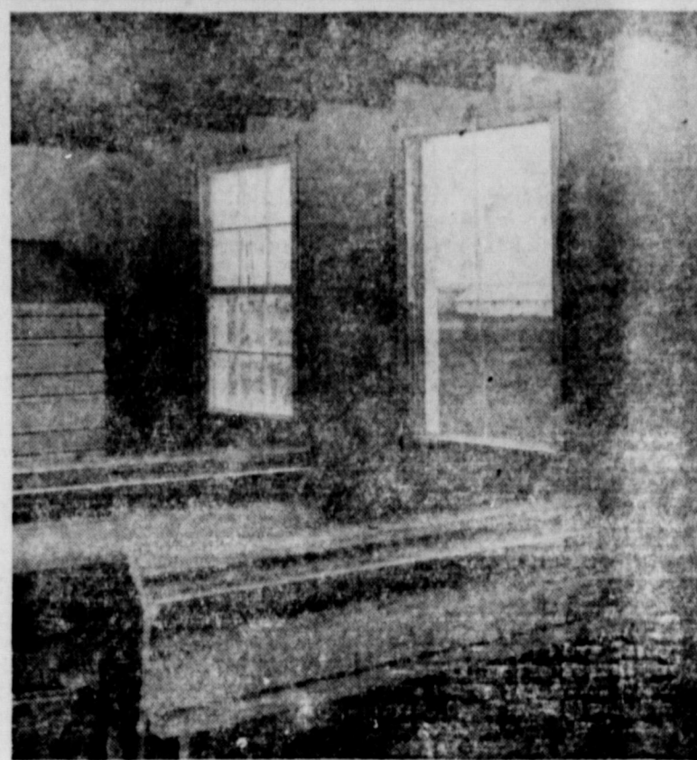
Added protection for the poultry flock now may be obtained through the use of improved building materials. The walls of this laying house, for example, have been lined with asbestos-cement flat sheets. These easily-applied sheets keep out rats and other rodents. They're peck-proof and fire resistant as well. Ease of cleaning helps promote sanitation and ward off poultry diseases.
